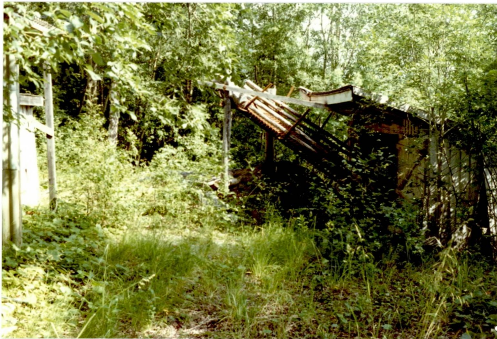
SUNNAN KALKBRUDD 1980. Rist for grovknuser.
