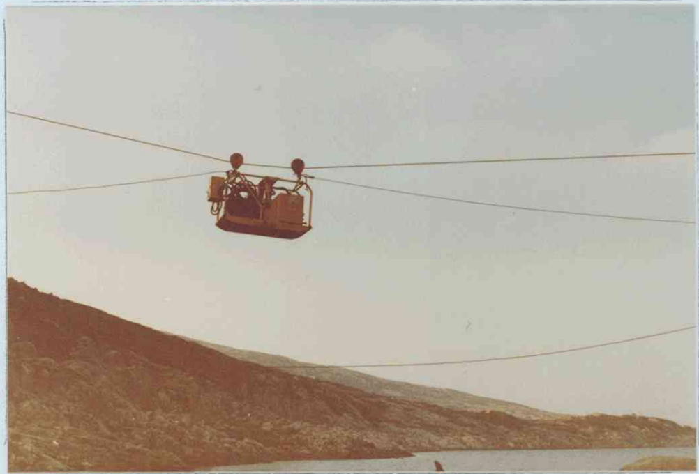
Winching the hydraulic aggregate (Diamec) across the Stutedalen valley to DH 4-84.
